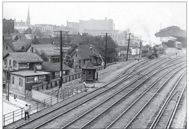
Demolition begins for the new Central Station, 1911 - 1912
