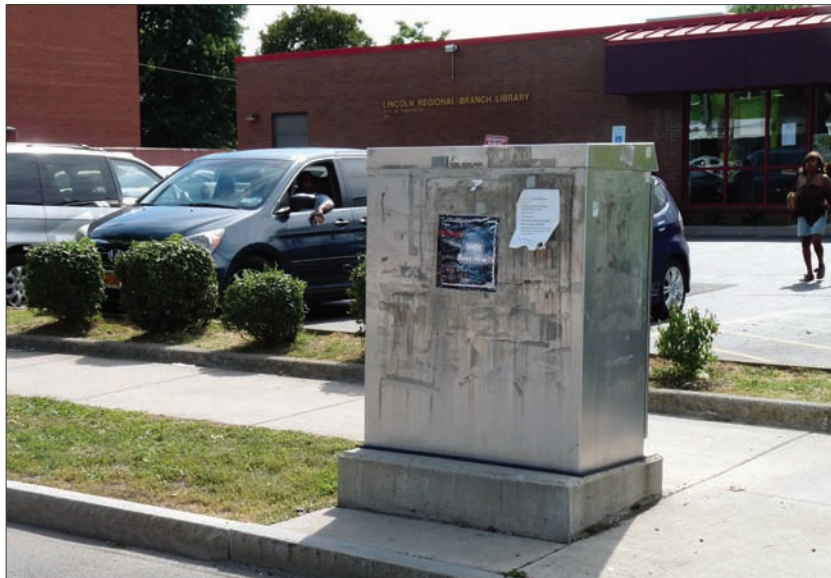
Traffic Switch Box - Before
