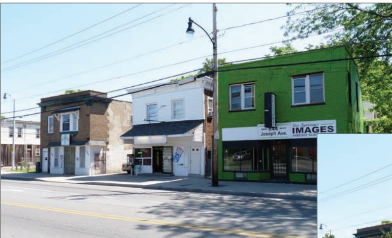
South of Avenue D - Before
